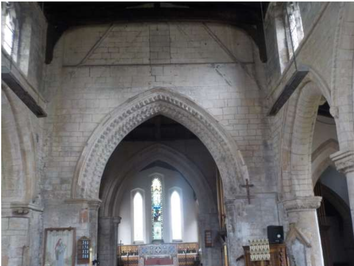
Figure 3 Crossing arch and indication of earlier roof line on tower wall.
