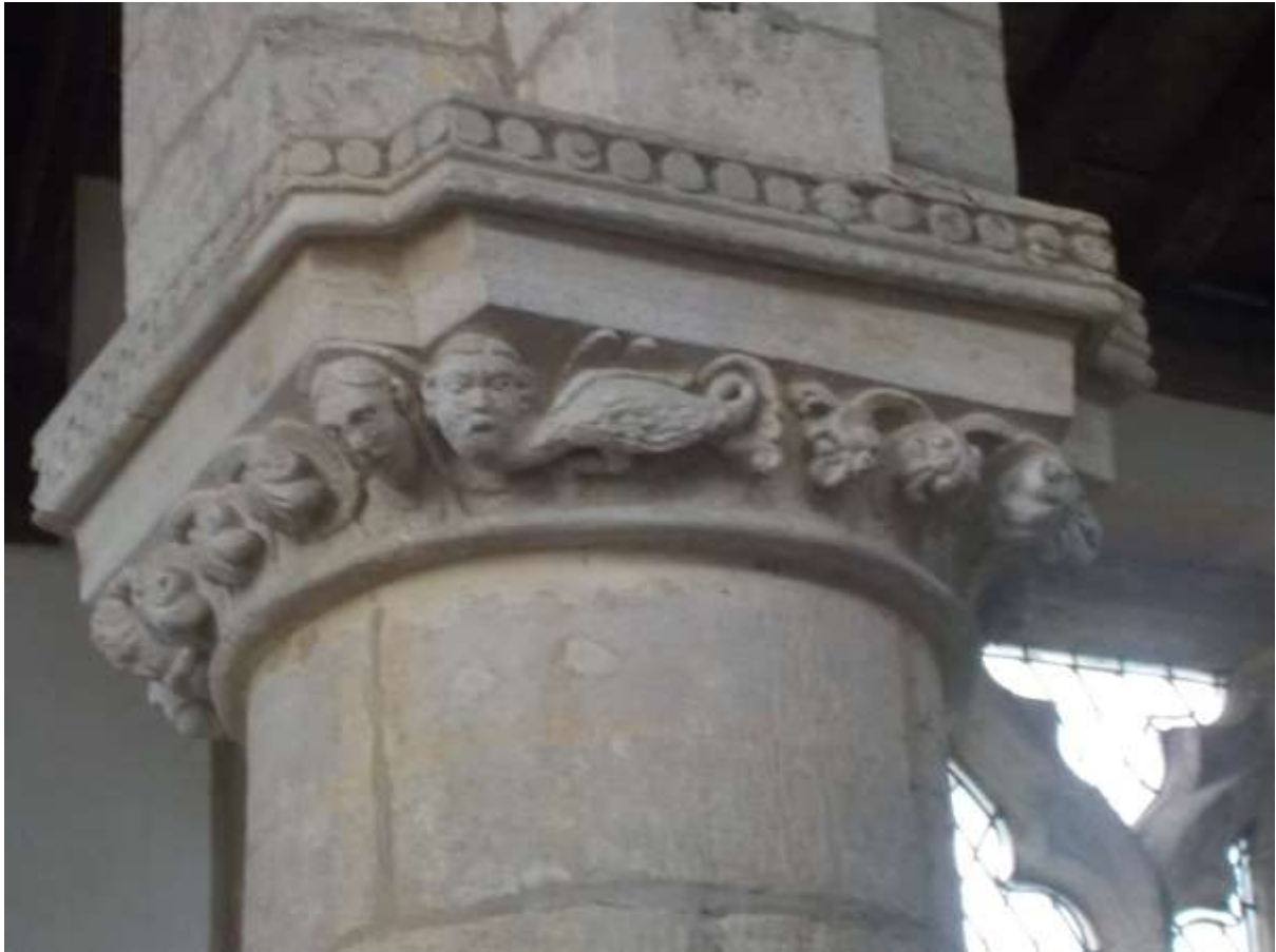
Figure 2 Pier capital, nave, north aisle.
